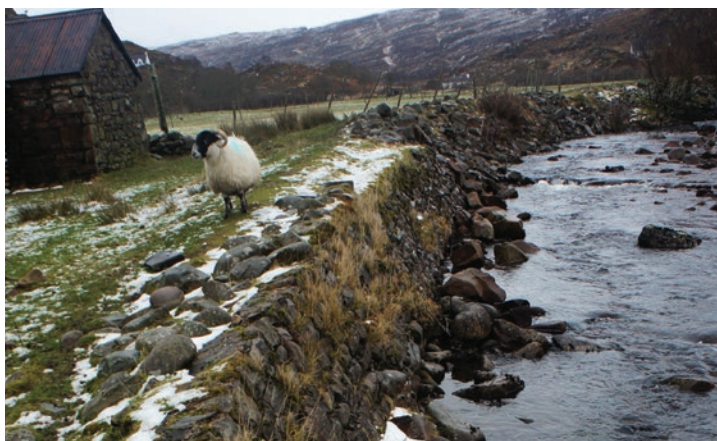
Reinforcement of the Toscaig River bank
